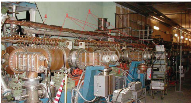
Figure 1: The existing INR DAW cavity. 1 – accelerating sections, 2 – bridge coupling cavities, 3 – RF input, 4- focusing elements.
