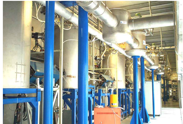
Figure 2: A view of ALPI high-energy branch. At centre one cryostat is missing for maintenance.
