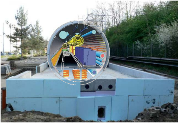
Figure 7: Picture of the tunnel mock-up at DESY. The final XFEL tunnel layout is included as a computer simulation.
