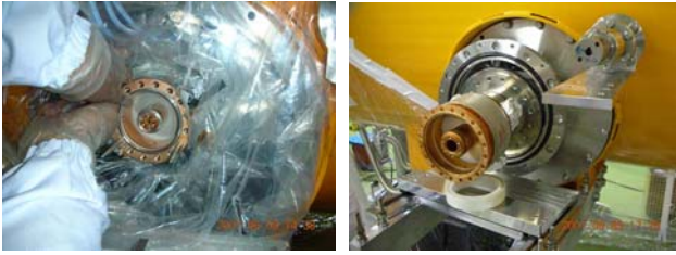
Figure 16: Installation of a warm coupler in a cryomodule.
