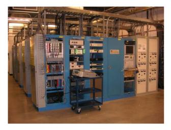
Figure 1: Layout of RF Amplifiers for Medium Beta Linac in the Power Supply Room
