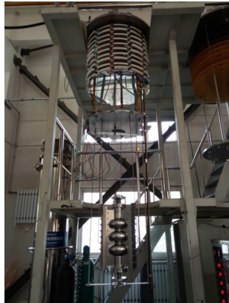
Figure 2: 1.3 GHz slotted cavity prepared for vertical test.
