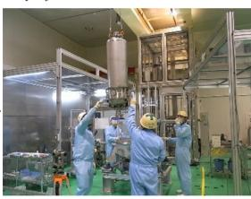
Figure 4: Heavy parts are brought into clean room using crane. Workers are wearing ISO7 clean ware and helmet.
