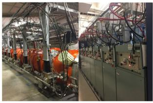
Figure 1: LCLS-II cryomodule in the LERF vault and four kW solid state amplifiers in the equipment gallery.
