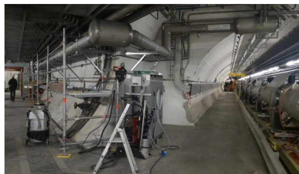
Figure 3: The cryogenic distribution line during installation in winter 2016-2017.
