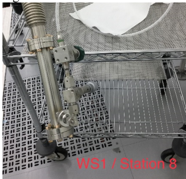
Figure 2: Nitrogen purging is relocated at the cavity side of corrugated vacuum hose.
