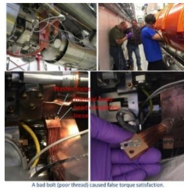
Figure 5: Thermal intercept repair.
