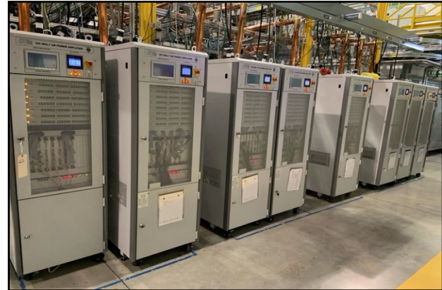
Figure 9: Eight RFPAs systems commissioned & coupled to SSR1 @ Fermilab.
