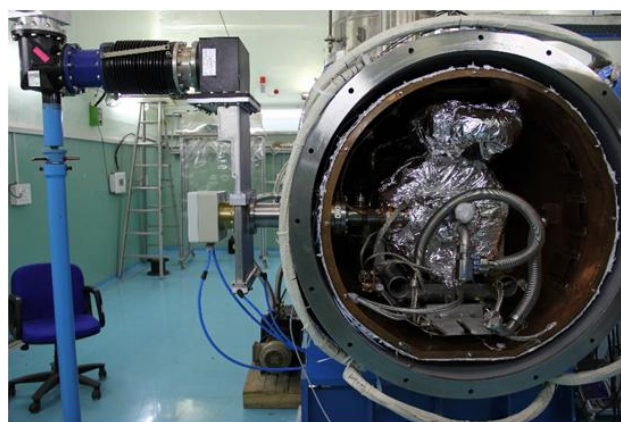
Figure 9: Dressed cavity with high power coupler (AES 10 from Fermilab) installed in the HTS cryostat at RRCAT.
